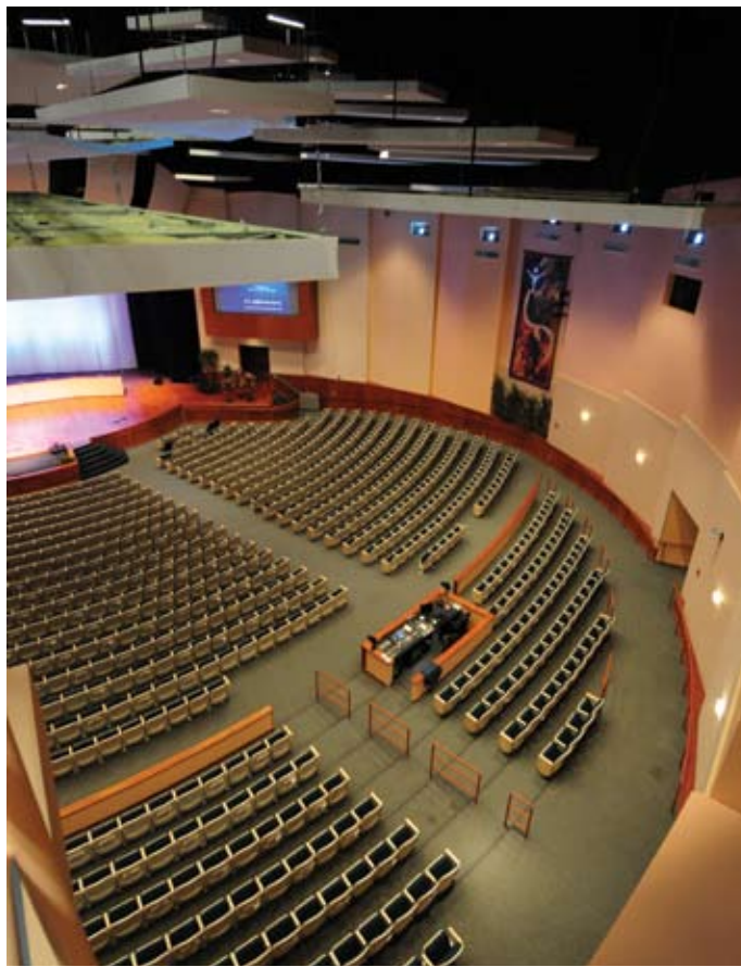
Acoustical clouds help keep sound from reverberating through the dome-shaped structure.
